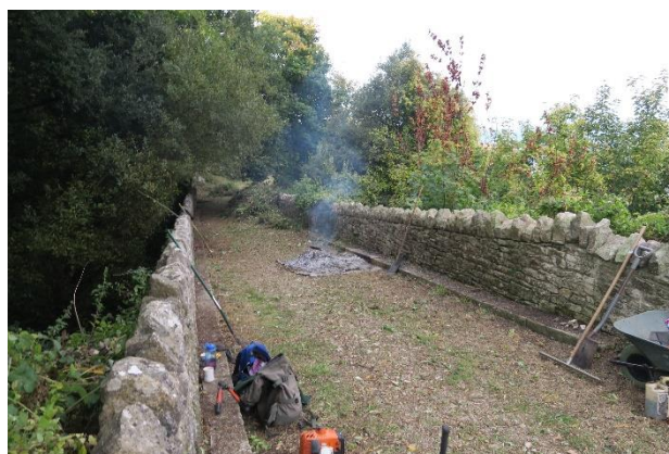
The bridge to Caravan Terrace
